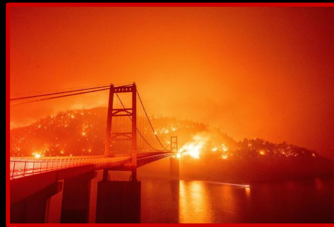
Bidwell Bar Bridge on September 9th 2020
